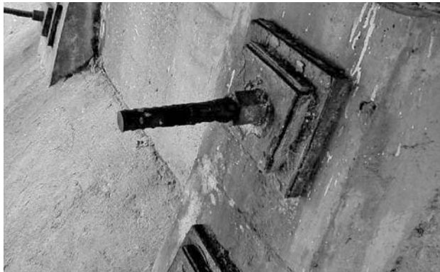
Figure 4.4 Anchor heads without protection
