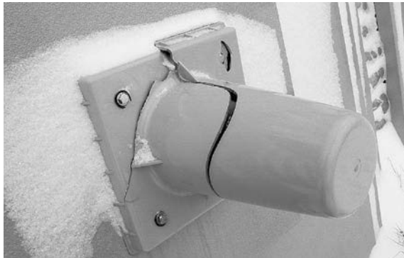
Figure 4.13 Damage to anchor cap caused by snow load
