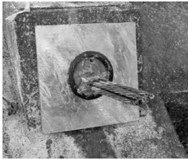
③ Fill below the bearing plate with corrosion inhibiting compound
