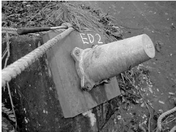
Figure 4.16 Leakage of corrosion inhibiting compound from anchor cap
