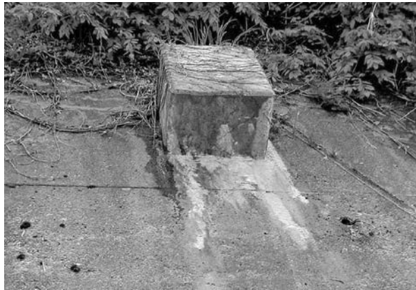
Figure 4.14 Lime deposits around anchor head
