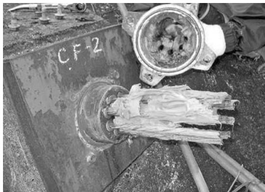
Figure 4.24 Deterioration of corrosion inhibiting compound (grease)
