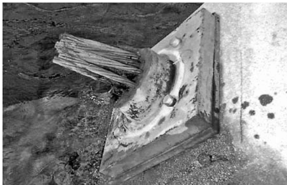
Figure 4.12 Damage to anchor cap caused by impact of rock fall or driftwood
