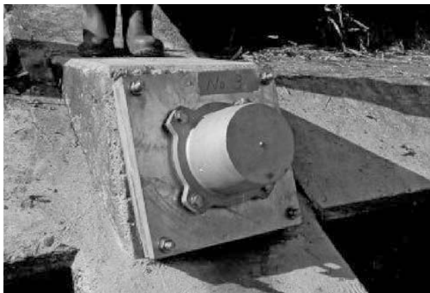
Figure 4.26 Protection by anchor cap after investigation
