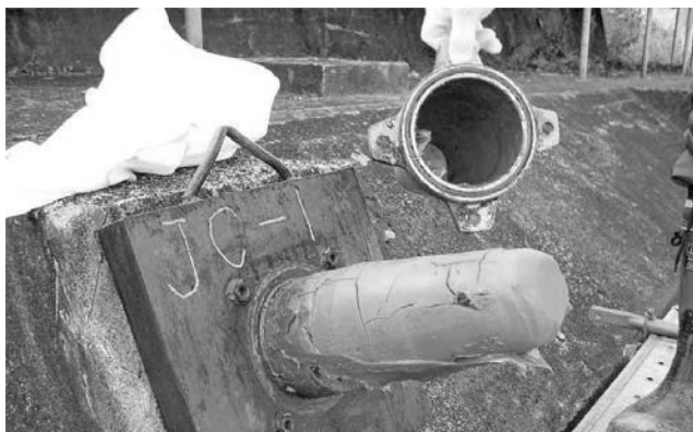
Figure 4.19 Filling of corrosion inhibiting compound
