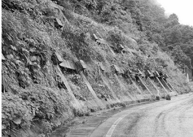
Figure 4.1 Anchor head with concrete cover
