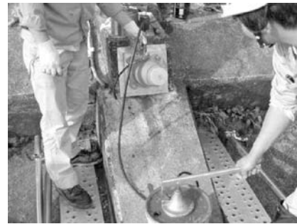
⑥ Filling corrosion inhibiting compound
