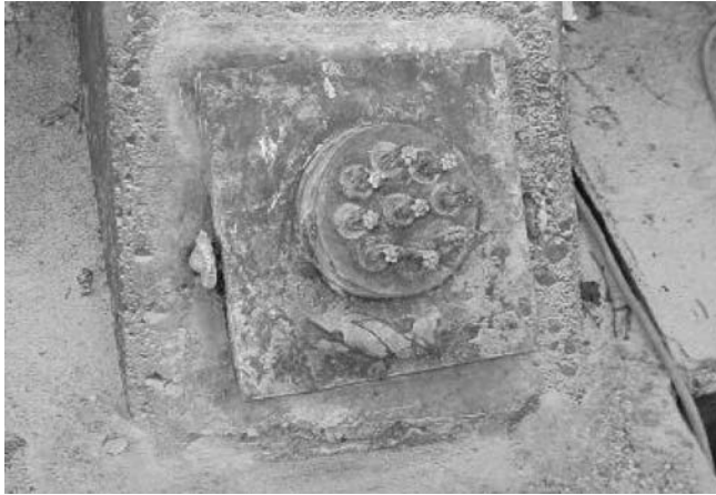
Figure 4.17 Exposure of a wedge type anchor head
