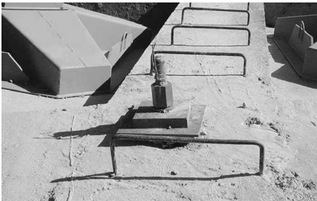
Figure 4.18 Exposure of a nut type anchor head
