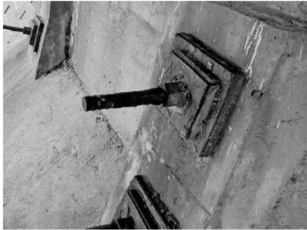
Figure 3.2 Anchors without anchor cap
