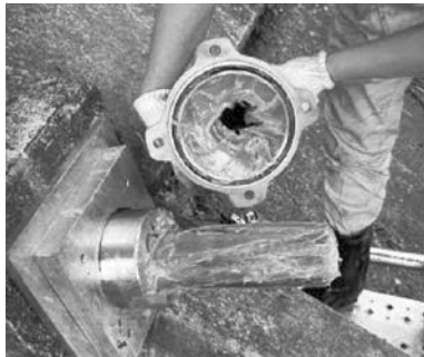
⑤ Fill anchor cap with corrosion inhibiting compound
