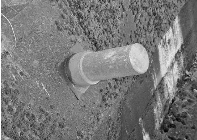
Figure 3.4 Simple anchor cap
