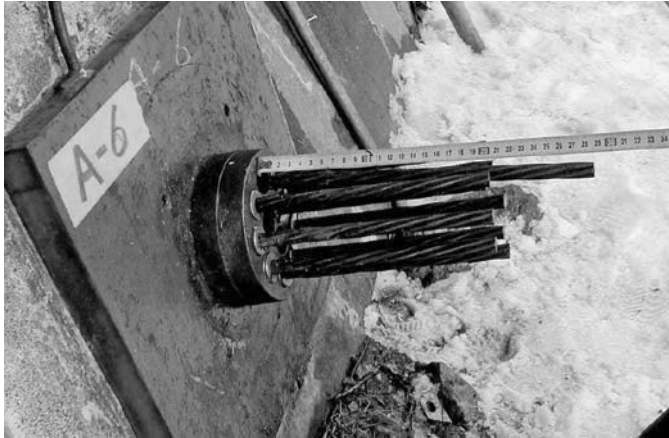
Figure 4.20 Irregularity of protruding lengths for restressing
