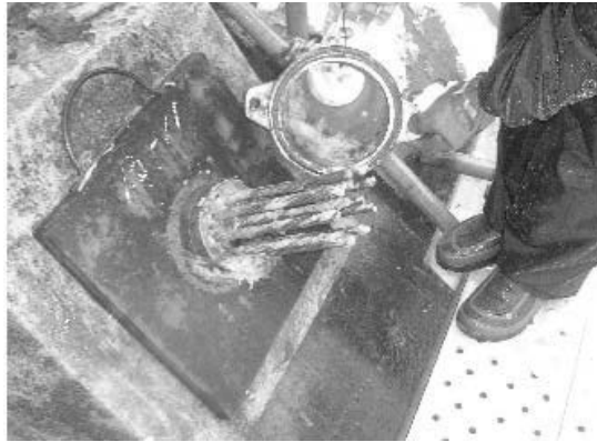
Figure 4.40 Corrosion inhibiting compound (grease) with colour change to turbid white or emulsion white
