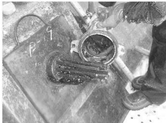
Figure 4.42 Corrosion inhibiting compound (grease) with colour change to black
