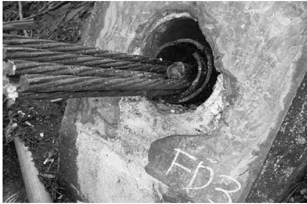
Figure 4.35 Trace of lime deposits
