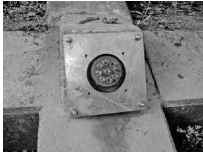
④ Setting plate for anchor cap
