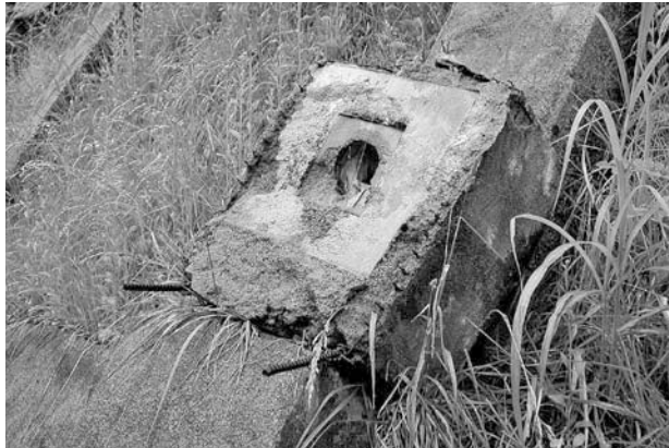
Figure 4.9 Dropping-off of concrete cover by frost heave
