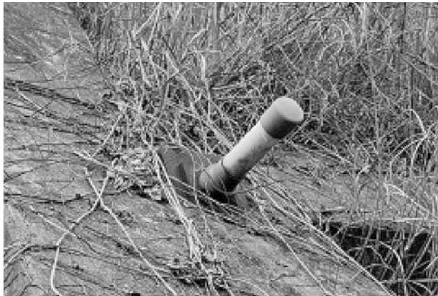
Figure 4.3 Simple protection of anchor head with pvc pipe
