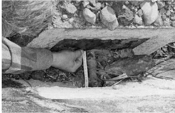
Figure 4.6 Damage by deformation of anchor (Failure of tendon below the anchor head)
