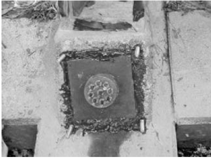
① Setting hole-in anchor
