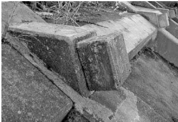
Figure 4.25 Concrete cover before investigation
