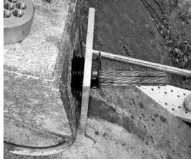
② Installation of materials for corrosion protection below the bearing plate
