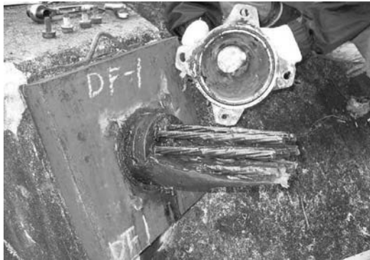
Figure 4.23 Leakage of corrosion inhibiting compound (grease)
