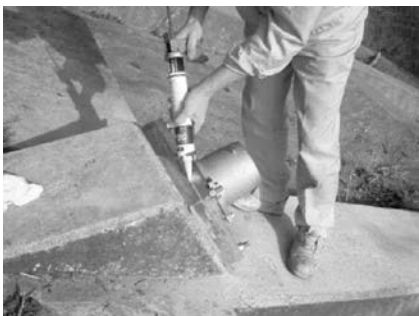
⑦ Sealing around anchor head
