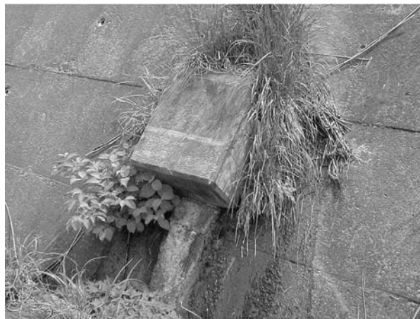
Figure 4.15 Groundwater leaking from below anchor head and abundance of weed growth
