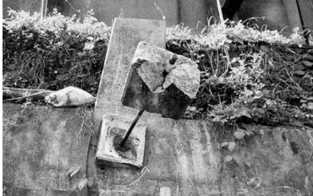
Figure 4.5 Damage by deformation of anchor (rupture of tendon in deep position of free length)
