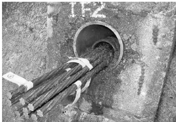
Figure 4.34 Ingress of soil and sand
