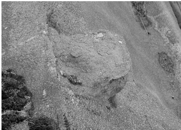
Figure 4.10 Deterioration of concrete cover
