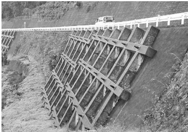
Figure 4.2 Anchor head with anchor cap
