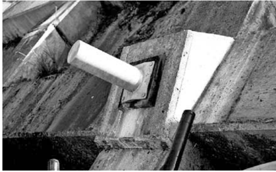
Figure 4.11 Deformation of anchor cap flange caused by rupture of tendon
